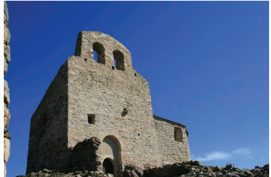
Restored Saint Etienne
