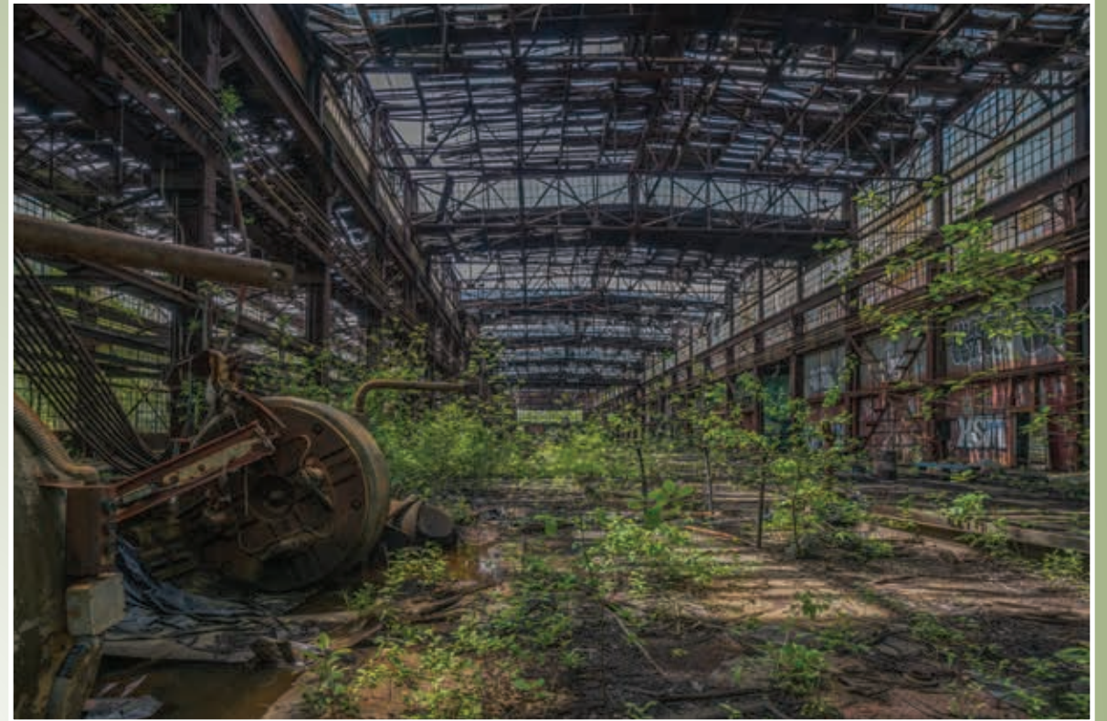
All the Iron Horses, Repair Facility
